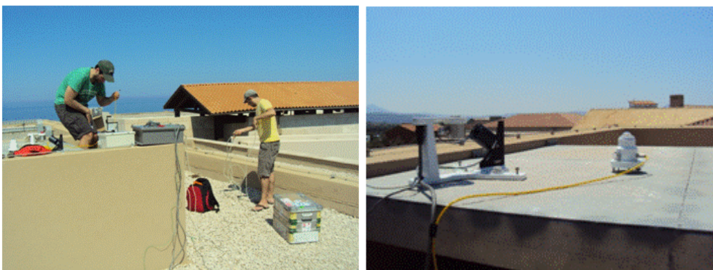
Figure 3. Installation works at the Luxury Romanos Hotel Reception roof.
